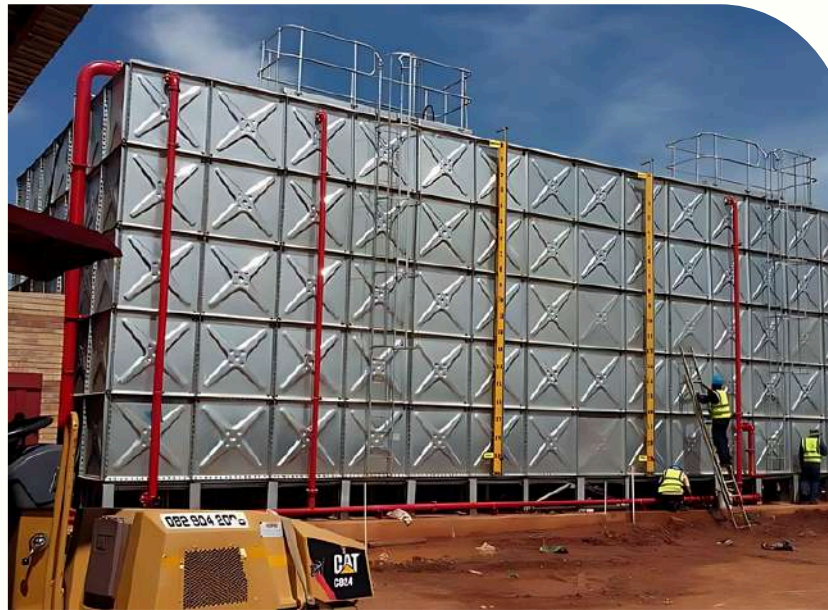
Galvanised Steel Water Tank Repairs
